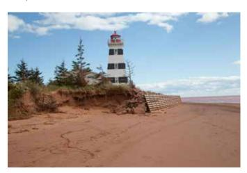
Figure 33. End-scouring on Langley Sea Wall at West Point (D. Jardine, 2019)
