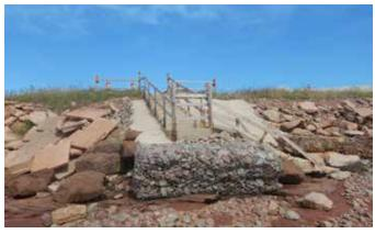
Figure 67. Beach access reinforced with poured concrete, concrete slabs and gabion baskets (H. Parnham, 2018)
