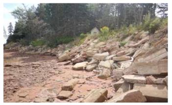
Figure 68. Typical residential shoreline armouring with old concrete/construction debris (H. Parnham, 2018)
